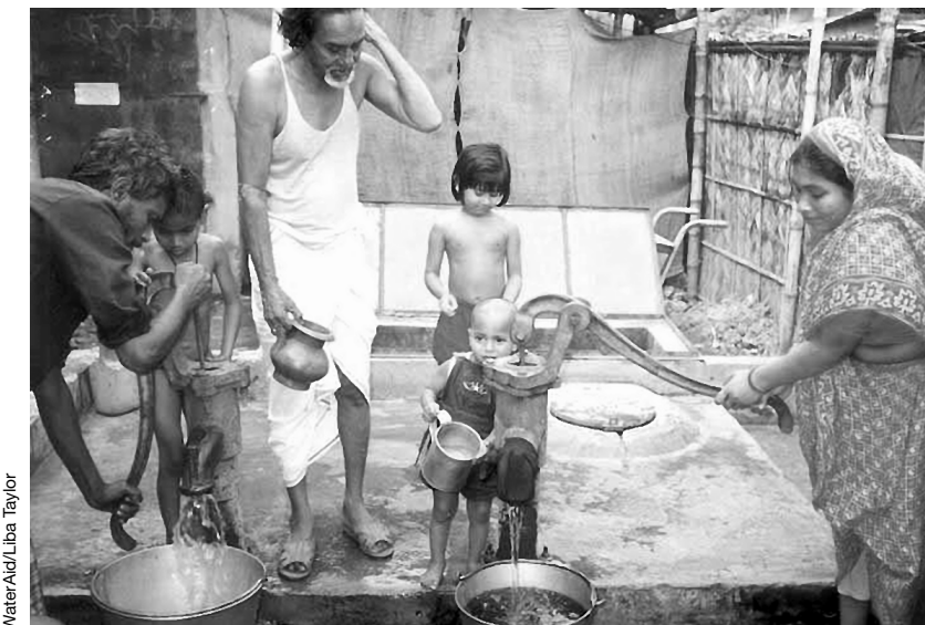
Photo 1: Water points consist of an underground storage reservoir, two hand-operated pumps and space for bathing and laundry
